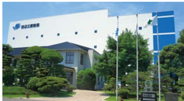
New pharmaceutical production building at the Yoshitomi Plant
