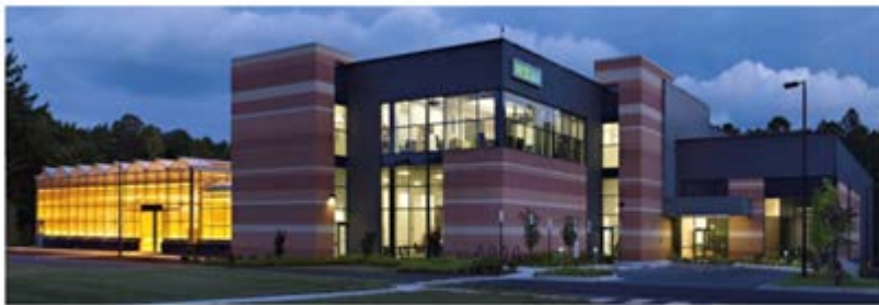
Commercial scale facility (RTP, North Carolina, USA)
