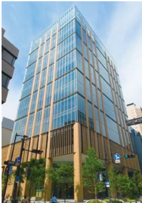
Exterior view of new Head Office building
