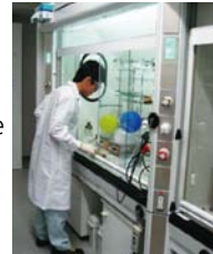
High-efficiency local exhaust ventilation system
