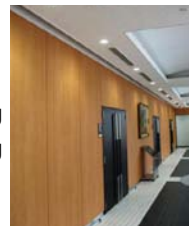
Use of LED lighting in hallways
