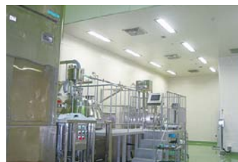
The Kashima Office after renovations were completed
