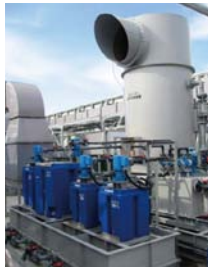
Air ventilation system
