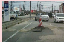
Manhole cover displaced by liquefaction of the ground near the Kashima Plant
