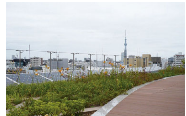
Rooftop solar panels
