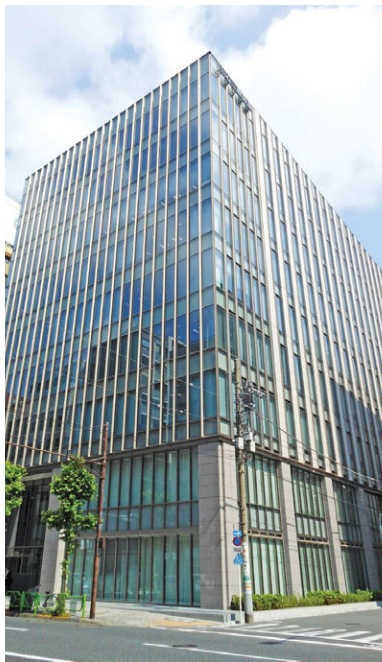
New Tokyo Head Office building
