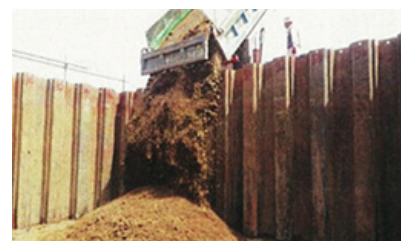
Soil improvement work at the former Kashima Plant
