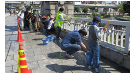
Working hard to clean the bridge railings
