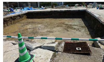
Soil Improvement at Yoshitomi Plant
