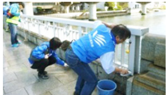
Working hard to clean the bridge railings
