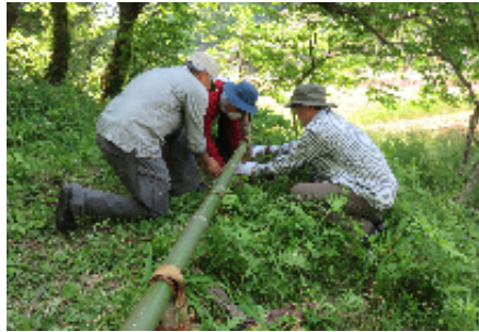
Making a bamboo fence
