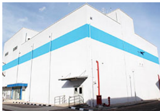
Mitsubishi Tanabe Indonesia Exterior view of new pharmaceutical production building
