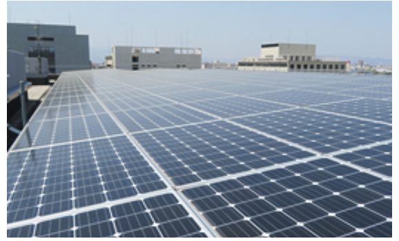
Solar panels on the roof of the Kashima Site
