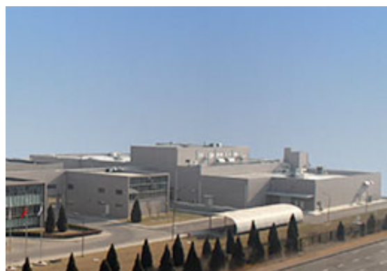
Tianjin Tanabe Seiyaku Exterior view of new pharmaceutical production building
