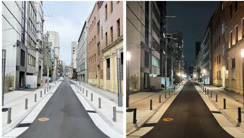
Road Maintenance from the Doshomachi Street Revitalization Project
