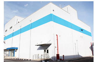
Exterior view of new pharmaceutical production building, Mitsubishi Tanabe Pharma Indonesia
