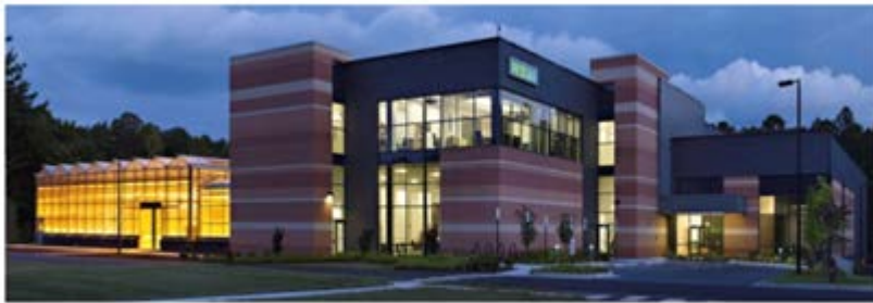
Commercial scale facility (RTP, North Carolina, USA)
